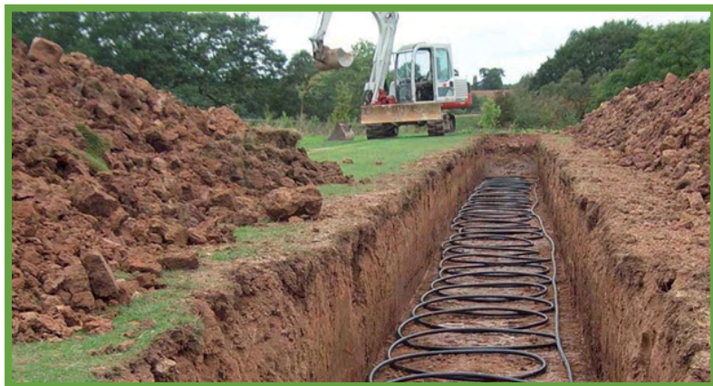
Figure 4.4: Horizontal Geothermal Installation
