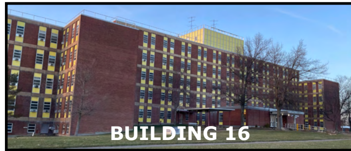
Figure 2.2: Main OPWDD Headquarters
