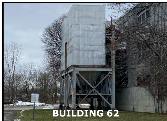
Figure 2.5: Former Laundry Building
